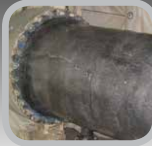
After Carbon Fiber Installation
