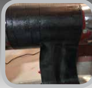
Carbon Fiber Installation
