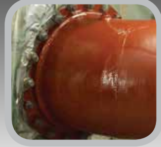
Final Repaired Pipe
